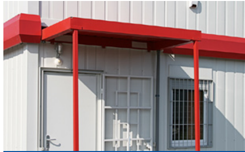
Canopy roof/ Fascia
