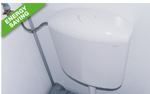
Flushing cistern with water saving device
