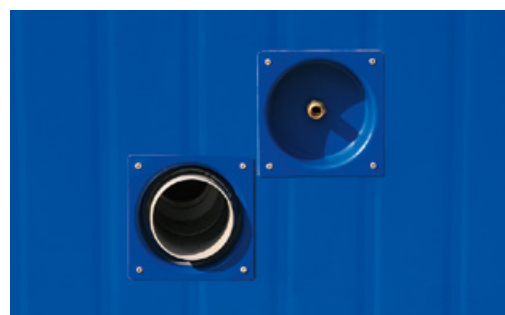
Water connection, embedded in the wall
