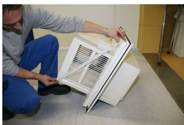
Position the A/C case at the top part of the frame (case should stick into the inside of the building by 21.5 cm from frame)
