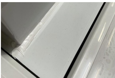
Use silicone to seal up the A/C case on all 4 sides of the frame
