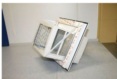
A/C unit fitted to the frame and ready for positioning
