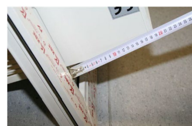
Position A/C case (case should be positioned 22cm to the inside of the container according to the drawing on page 4)
