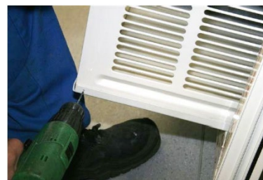
Drill and bolt braces to A/C support
