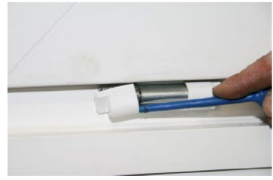
Removal of hinge covers
