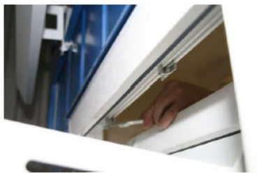
Fix window fitting
