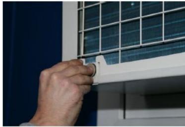
Fit condenser pipe to the outside
