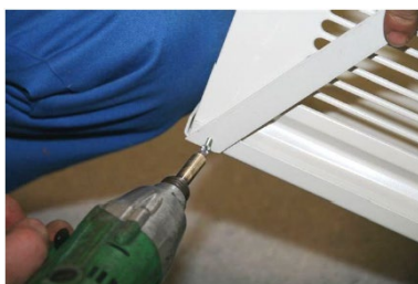
Bolt A/C case to frame
