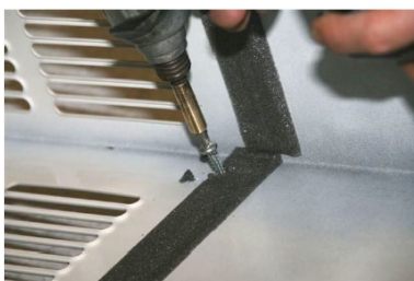
Bolt A/C case to frame
