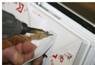
Bolt 2 braces on the left and right side to the frame
