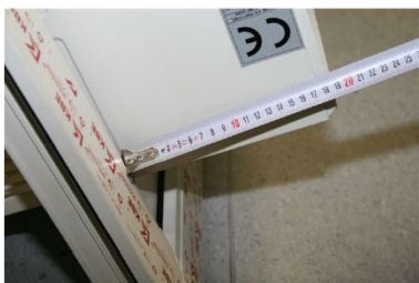
Position the A/C case at the top part of the frame (case should stick into the inside of the building by 21.5 cm from frame)
