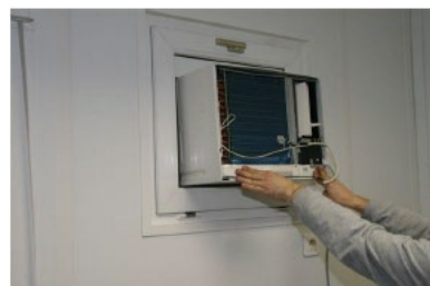
Fit fixing clamps
